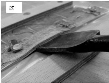
Use a pad under the hammer when pulling the nails. If a nail head breaks off, use vice grips (pull straight up & twist) to pull the nail out. PHOTO 21
