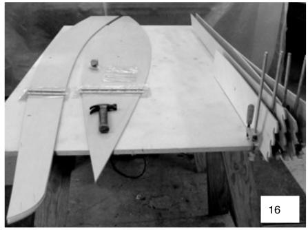
**Panels 2 next.** Don't forget all 3 layers of plastic and the nails that hold the edges flush. PHOTO 17
