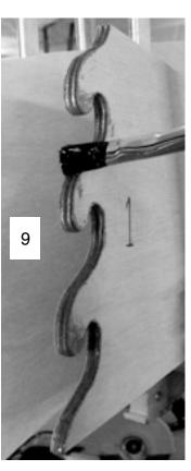
Place plastic over the joint before fitting the next layer of panel 1. PHOTOS 12 & 13
