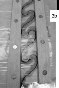
Pre-cut strips of plywood are placed either side of the puzzle joints. Nails are driven through into the bench to pull the joints flat when gluing. PHOTOS 3 & 3b
