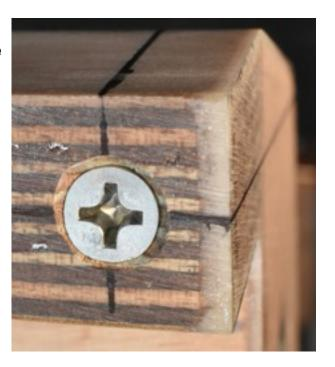
Set the hull-halves on edge leaning against the bench as shown to put gravity to work. Both sides can be done with one batch of un-thickened epoxy. **Pinch the cup and pour epoxy down one edge of the holes until they are full.** Use a piece of wire or skinny long
