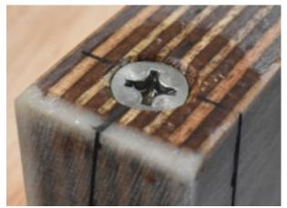
With the holes full of epoxy, drive the screws.
