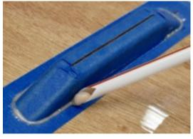
Clean-up is best done with a plastic straw with the tip snipped off at 45 degrees.
