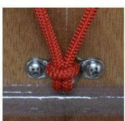
We used 3/16" line for the handle, held with stopper knots (photo on right) and 3/16" shock chord (both photos) for the bailer holder.
