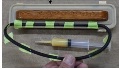
Each end can be lifted, glued, and taped back down. Remember to place a piece of tape over the glued butt joint before dogging the cap back down.
