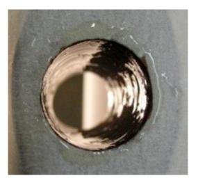
Mount the sockets dry with the 5/8" #10 screws. Remove and fill the screw holes with **un-thickened epoxy** with the tip of a small nail or something similar.
