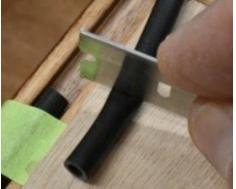
Expose more than half of the gasket notch as shown below.
