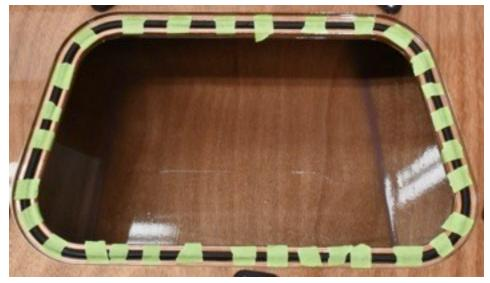
Tightly tape over the tip of the syringe and push the air out to make it last. The remaining gasket can be glued much later the same day, or the following day.
