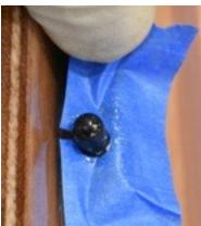
Just don't forget to carefully wipe up the excess and pull the tape. The slit in the tape will allow pulling the tape without wiggling the stops.
