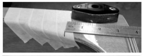
The pads that cover the gusset tips are easier to install.
